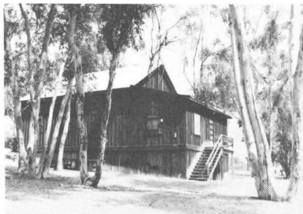
The 1916 addition is clearly defined from the original meeting hall by the stepped roof lines.
