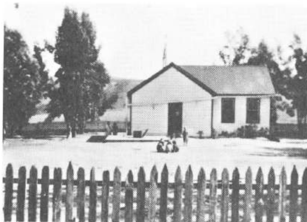
West side of Olivenhain school. Cistern is now directly under the house at 2365 7th Street.
